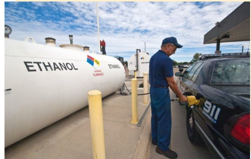
Image: NREL Image Gallery #18090
