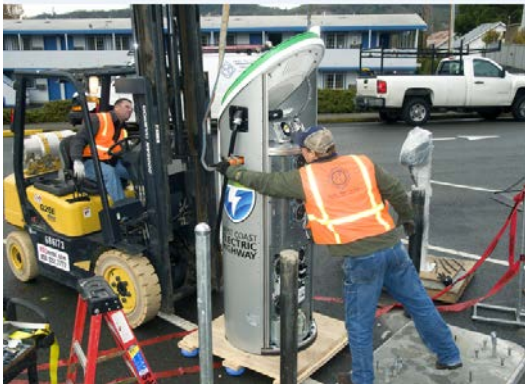
WCEH Charging Station Construction
