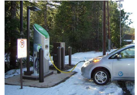
Mount Hood WCEH Charging Station
