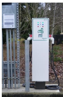
EV Charging Station
