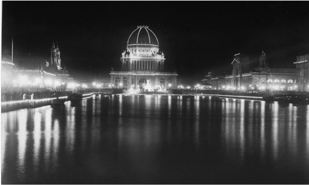
1893 Chicago World's Fair "White City" showed the potential of electrification
